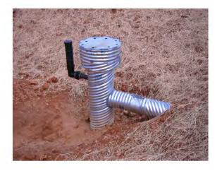
Figure 7.31-6 Dewatering device on Riser with Trash Rack
