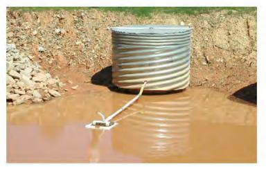
Figure 7.31-10B Floating Skimmer Installation
