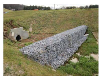
Figure 7.31-2C Forebay with Porous Berm (Gabion Rock)
